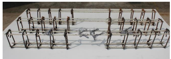
Fig. 3 A view of GFRP reinforcement cages
